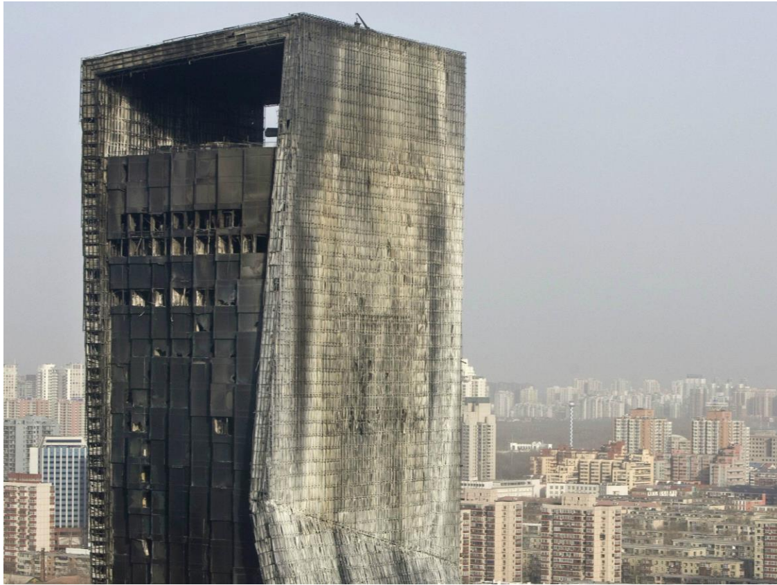
TVCC Tower, PRC 2009
